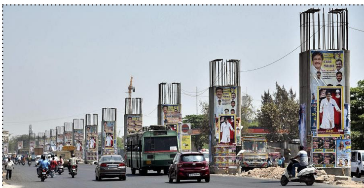
Maduravoyal elevated corridor
