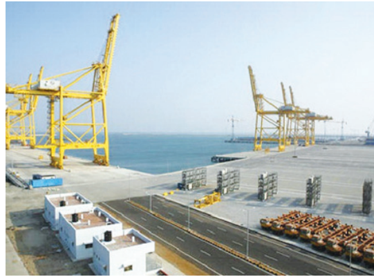
Kattupalli port; one of 'the Mega ports run by private institutions'
