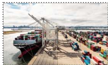
Pic: Port of Oakland
