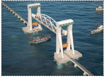
New Pamban Bridge
