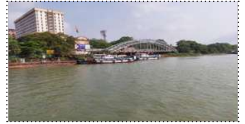
Jetty on the bank of Ganga
