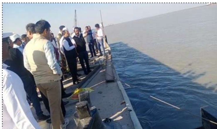
Work of Kandla's Liquid Jetty No 7 in final stage
