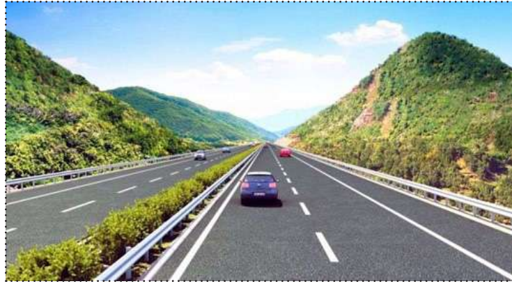
Char Dham expressway
