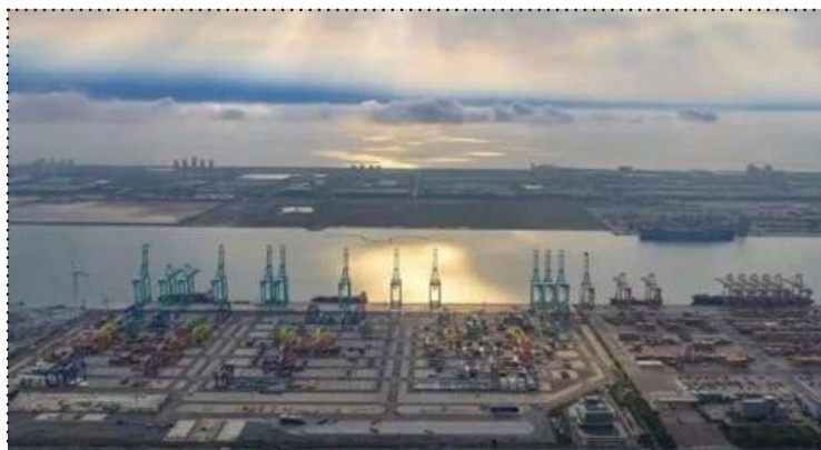
One of the five wind turbines is visible at the left side of the photo (Tianjin port COSCO)
