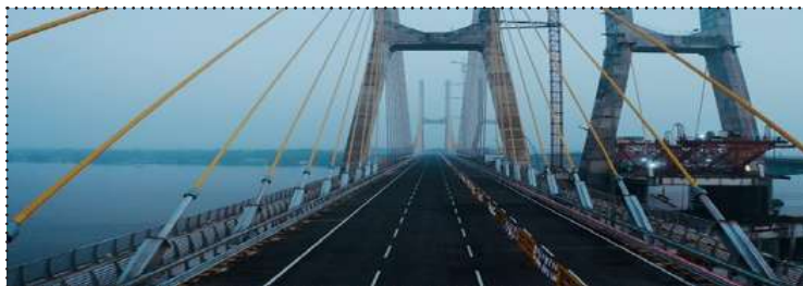
Zuari Bridge in Goa
