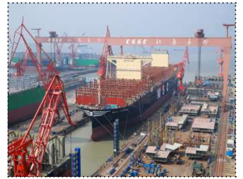
MSC Tessa under construction at Hudong-Zhonghua Shipbuilding. With a carrying capacity of 24,116 TEU, MSC Tessa will surpass Evergreen's Ever Alot by 112 TEU to take the title of world's largest Con.
