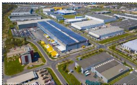
Multimodal logistics park
