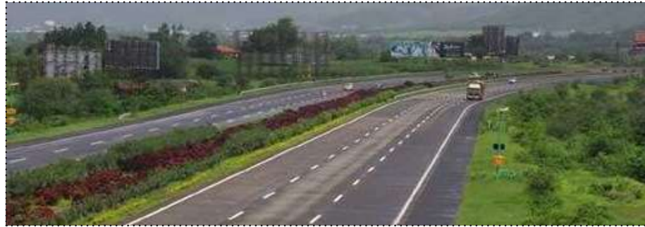
Chennai Bengaluru Expressway
