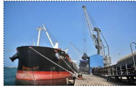
Tk 600 cr invested to construct 6 jetties on Karnaphuli river
