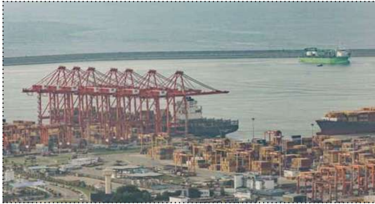
Galathea Bay Transshipment port on the Nicobar Islands, scheduled to be commissioned by 2028 according to an official release
