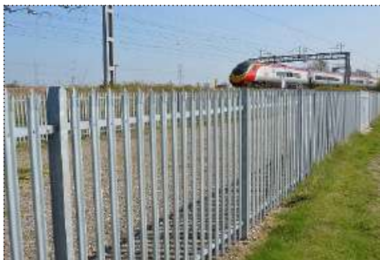
Picture of fencing of railway track a representational picture
