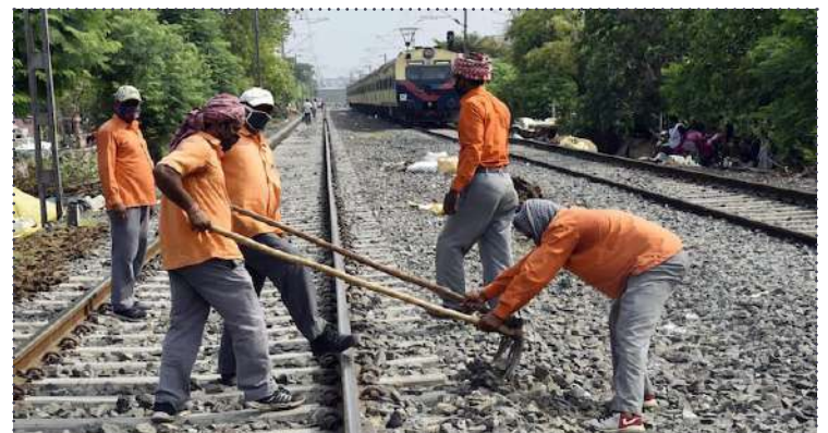
Railway track doubling
